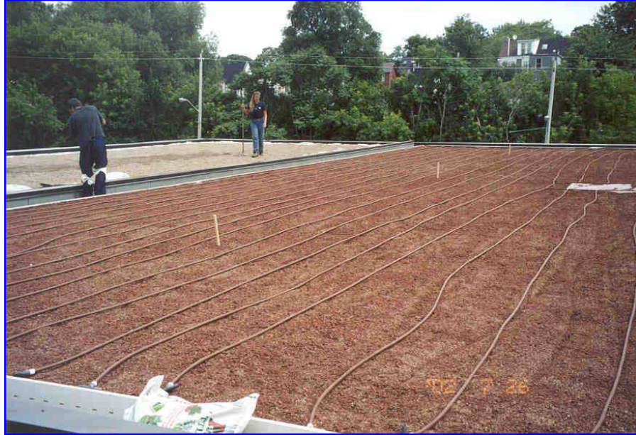
Figure 1: Growing Medium and Irrigation System Being Installed on the Roof of the Eastview Neighbourhood Community Centre
